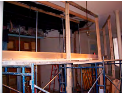
Recital Hall under repair
